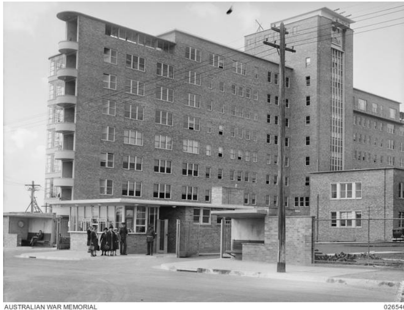
The entrance to 113 AGH Concord shortly after its completion in 1942. (AWM 026546)
