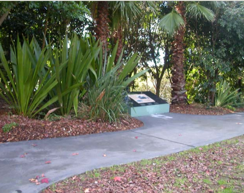
Newly concreted pathway.
